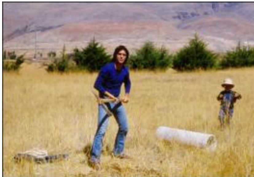
Fig. 10: Preparation of the base to install the cylindrical concrete pedestal.
