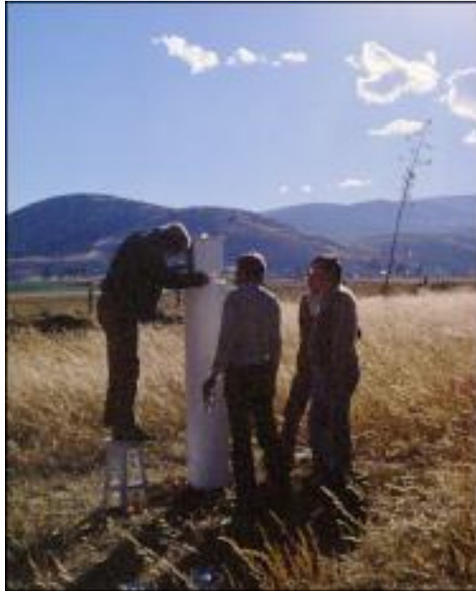
Fig. 11: Final installation of the pyranometer on the cylindrical pedestal.
